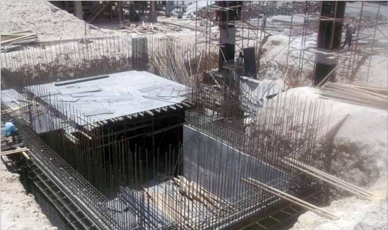
The gypsum crusher was challenging to design because half of the building is underground. The structure above ground is made of steel while the underground structure is made of concrete.
