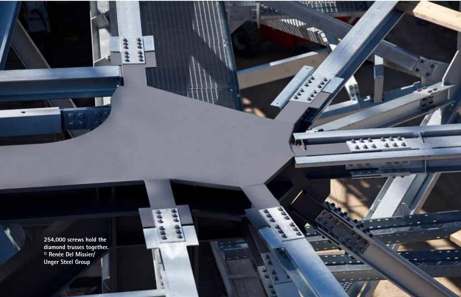
254,000 screws hold the diamond trusses together.
